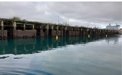
C: Western Wharf, looking northwest
