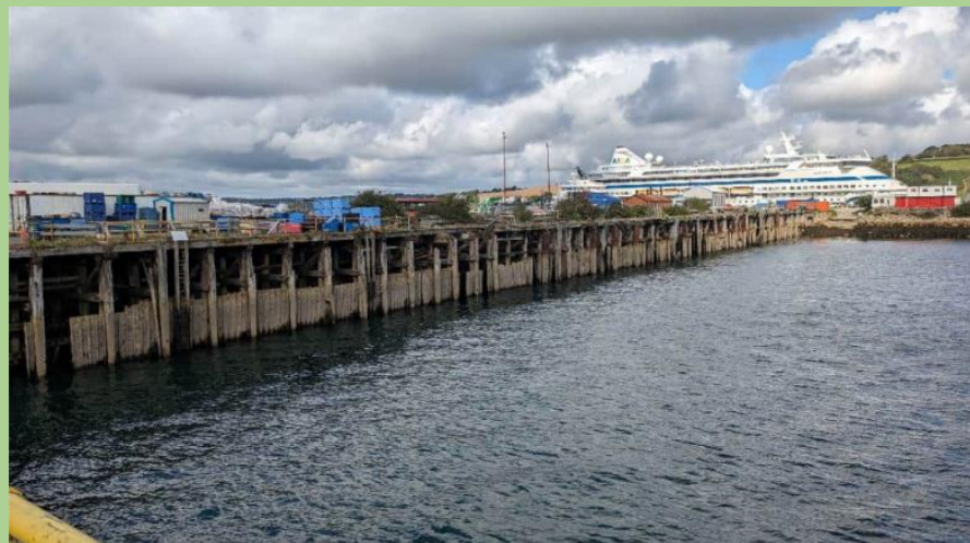
Photograph of existing causeway, taken south-east of the causeway, facing north-west
